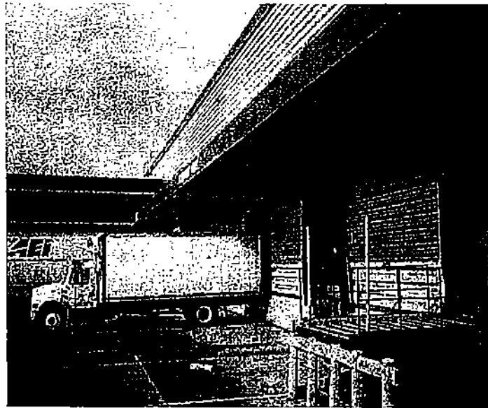
Figure 1 - Covered loading dock.
